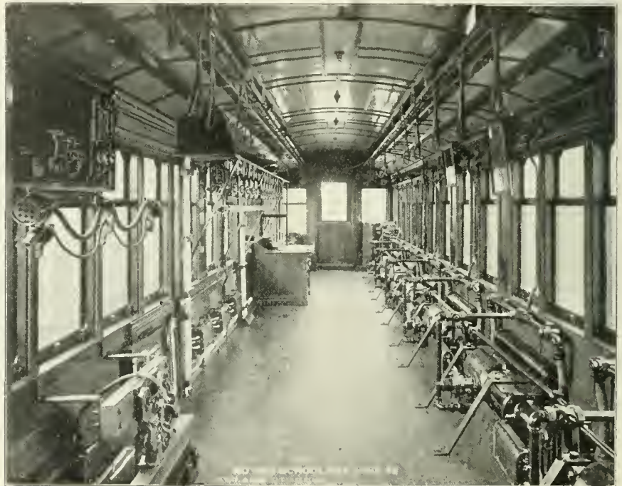
INSTRUCTION CAR, NEW YORK "L." AIR AND ELECTRICAL EQUIPMENT.
